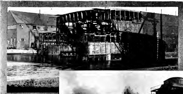
Forward section of the steamer "Sir Trevor Dawson" ready for launching, Sept. 9, 1916, and in drydock at Superior, Wisconsin, ready to be built onto the after section of the steamer "Moreland."
